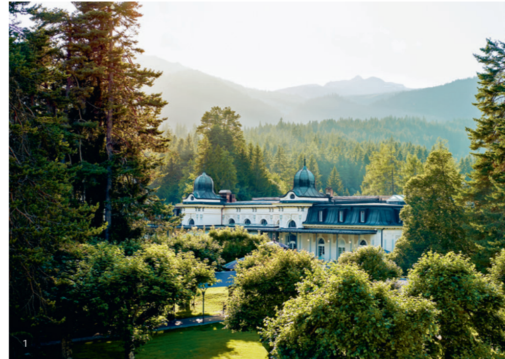
1 “Belle Epoque” Pavilion, 2 Pavilion Terrace
